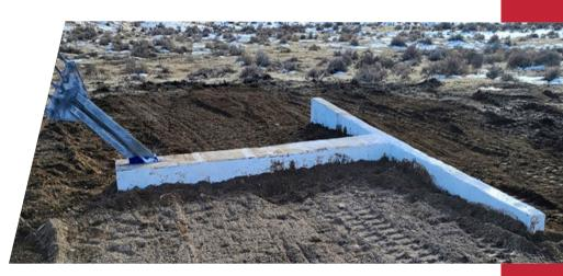
To address challenges with guy anchor corrosion while enhancing tower capacity, Congruex Engineering Services has developed the Guy-Lock<sup>™</sup> method, a patented solution that eliminates the need to disconnect guy wires, dig to the anchor block, or install a new anchorage point.
