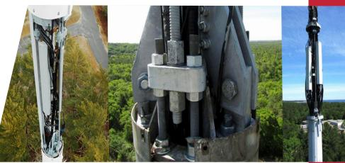
The patented Spine Saver<sup>™</sup> method for reinforcing Concealed Design Structures (CDS) avoids the need for full removal and replacement of the spine which prevents service interruption.
