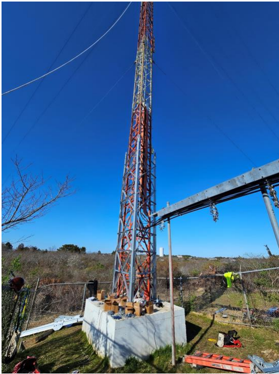
First sections of new tower being installed around existing tower
