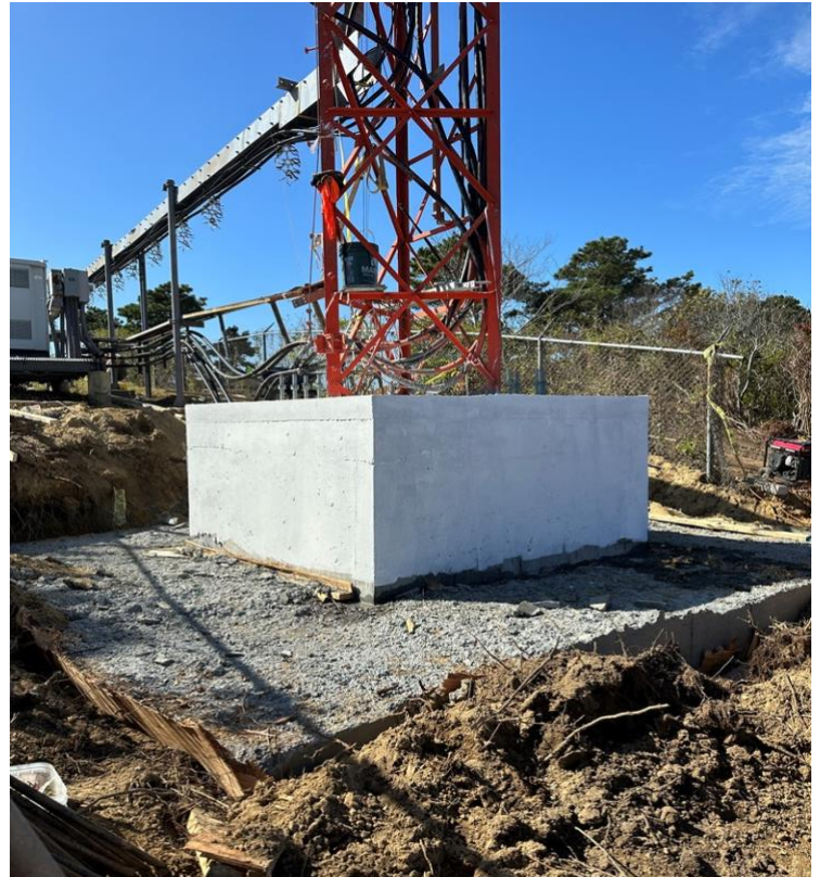
New tower base foundation installed encasing existing foundation
