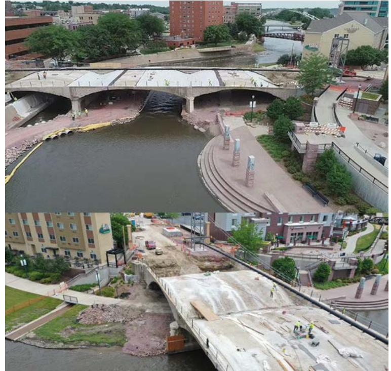
8 th St Bridge - Sioux Falls, SD
