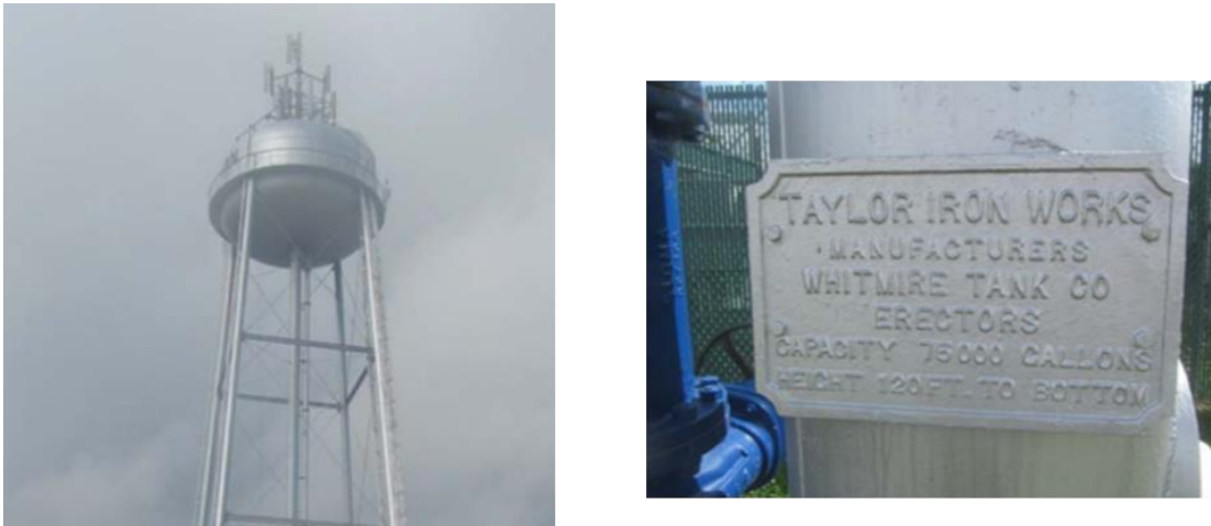
Figure 22. Images of water tank.
