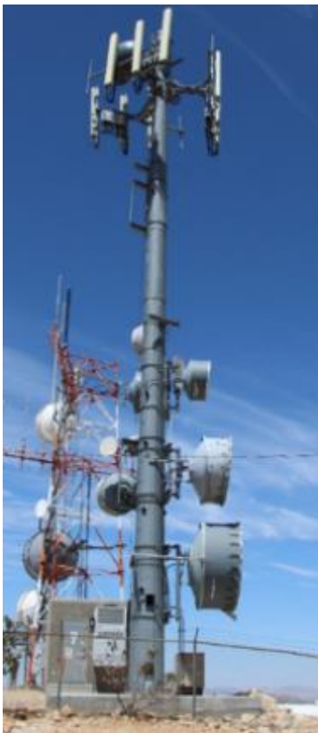
Figure 13. Image of a monopole
