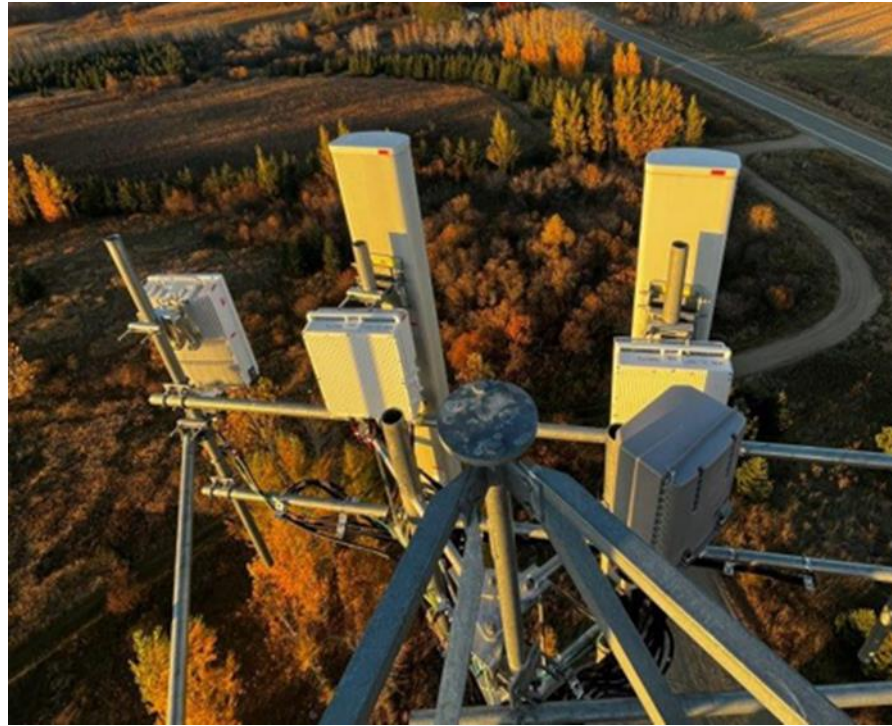
Figure 9. Image showing tiebacks attached to tower bracing, which introduce significant forces into tower members that are not designed to handle them. Multiple tower owners have prohibited this practice. In the example shown below, over 1300 lbs of potential force may go through the tieback.
