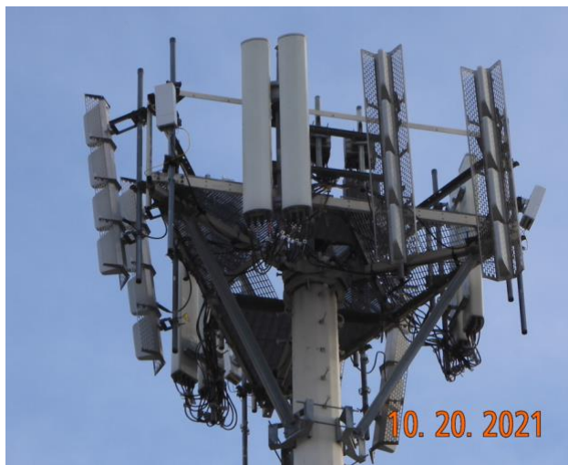
Figure 11. Images of mount components and/or equipment placed outside of the lease space. The photo on the left shows the mount initially installed with the new kicker kit. Because the kicker kit was not trimmed, it was installed ~3.5' below where it was proposed, putting the MNO tenant outside their contracted lease space. The photo on the right shows the final configuration after the EOR flagged the condition on a PMI and had the GC correct.
