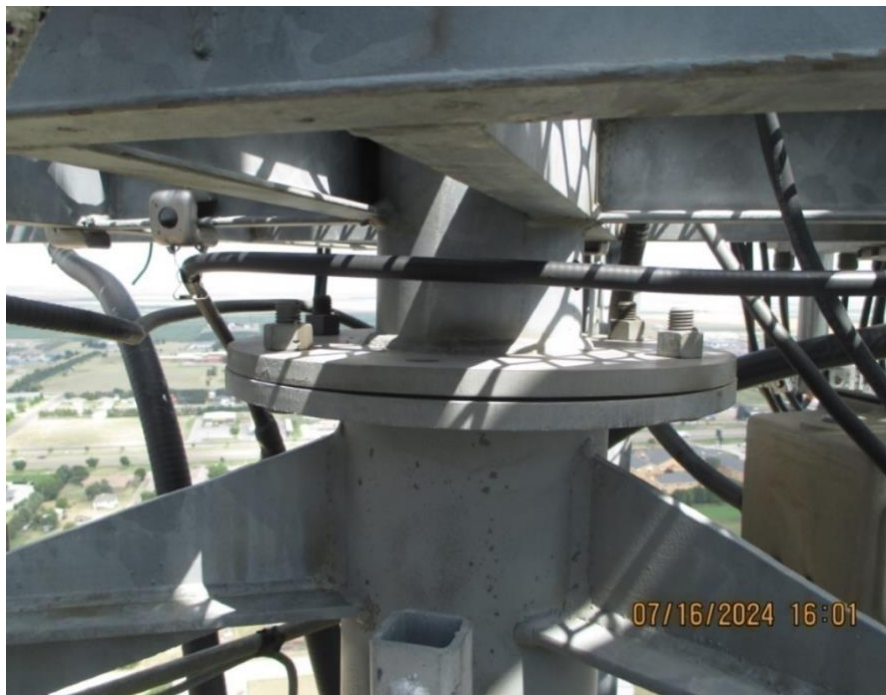
Figure 28. Image and illustration of mount-to-tower connection.
