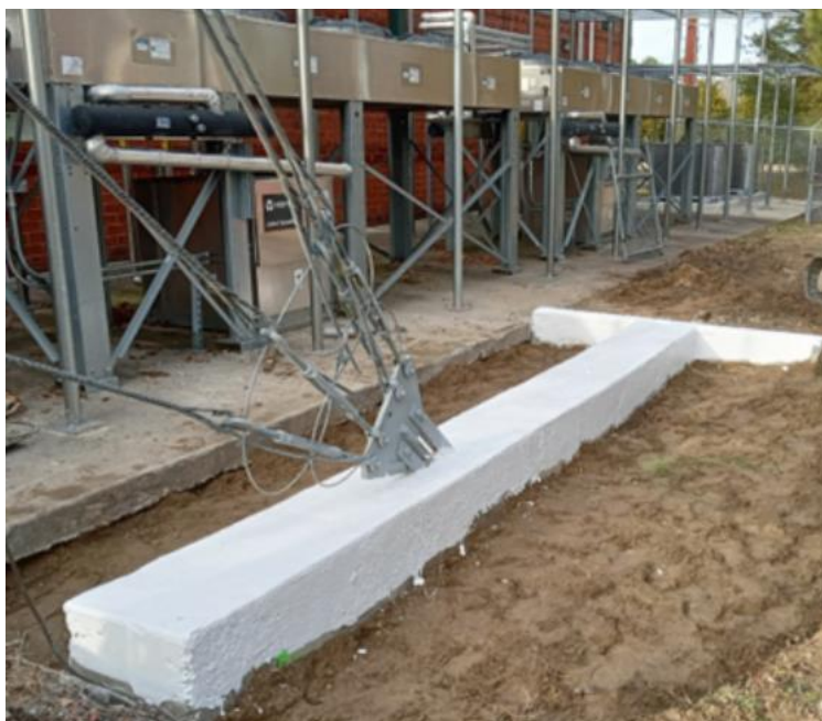
Figure 25. Image of Congruex's patented Guy-Lock™ solution [4]
