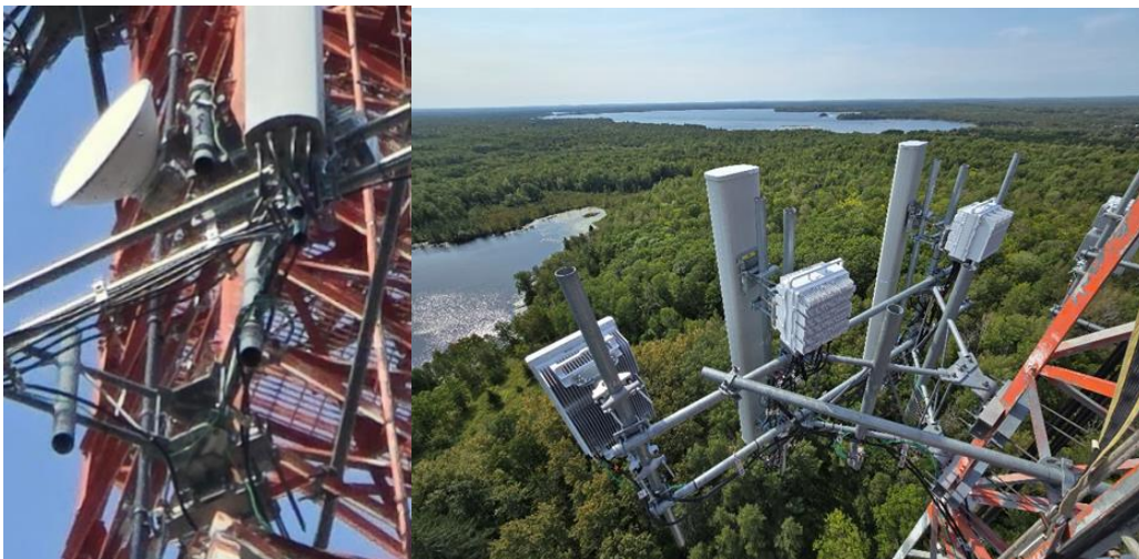
Figure 9. Image showing tiebacks attached to tower bracing, which introduce significant forces into tower members that are not designed to handle them. Multiple tower owners have prohibited this practice. In the example shown below, over 1300 lbs of potential force may go through the tieback.
