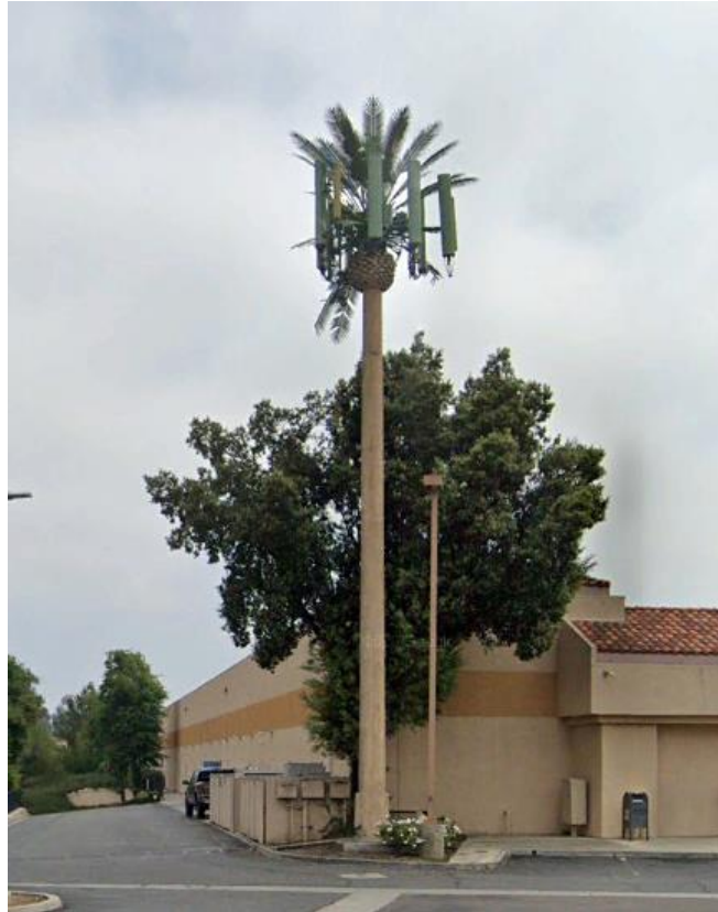
Figure 18. Image of a pole with reported overstress.
